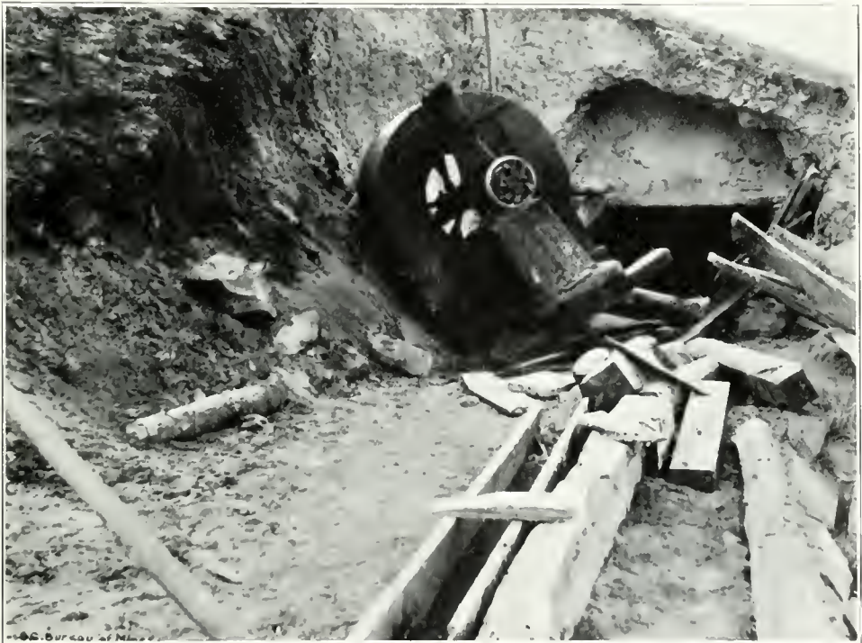
Diamond Vale Colliery—showing Fu as thrown by Explosion.
